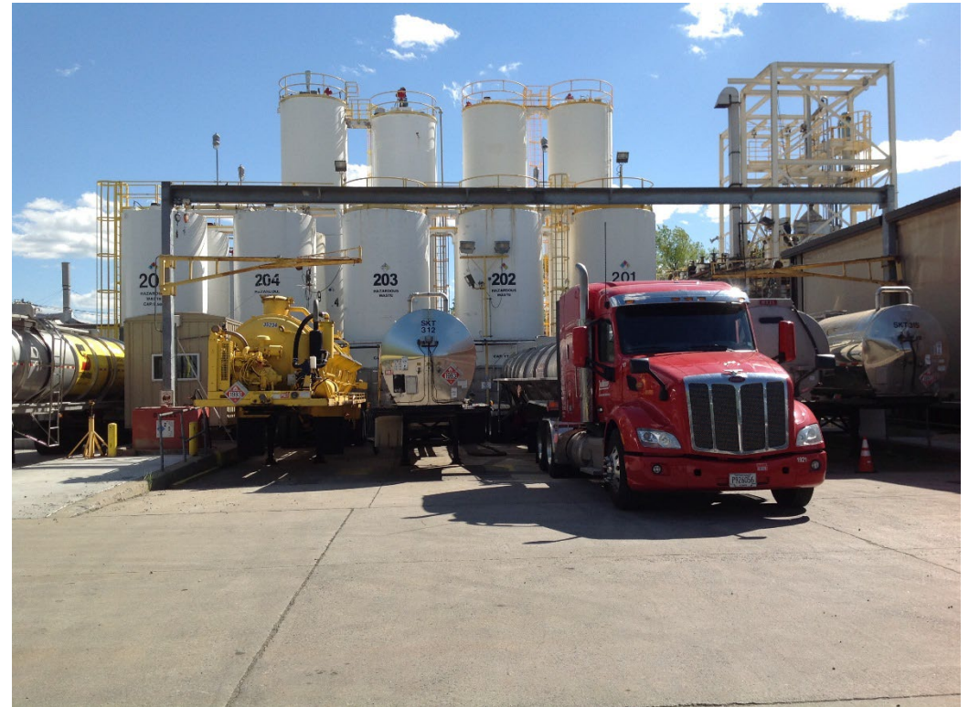
Photo 27 - Tank 2 (North Side)
