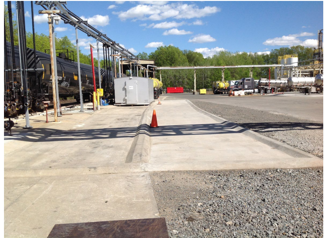
Photo 18 – Truck Stations 8, 8A, 9, 9A & 10 (West Side)
